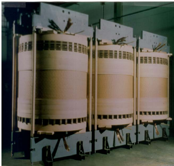
SMIT windings with individual phase clamping
